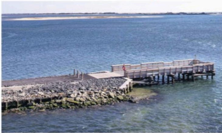
The recently renovated pier at Ponquogue Bridge is a prime fishing spot.
